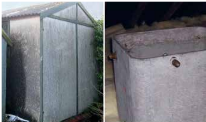
Asbestos cement panels and roof sheets / asbestos cement water tank
